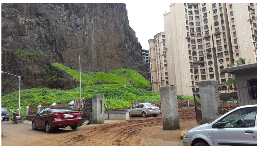
Fig. 9. : New construction at a very short distance from Gilbert hill
